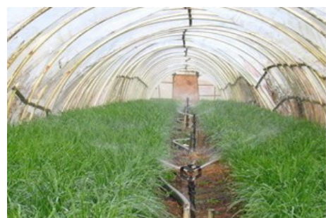
Agricultural greenhouse water supply system
